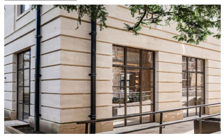
T60 innovatively combines the design and look of traditional hot rolled Crittall steel window profiles with contemporary materials to deliver an enhanced thermal barrier system. The cold formed steel frames retain the narrow sightlines and iconic profile providing maximum natural light and excellent thermal performance.
